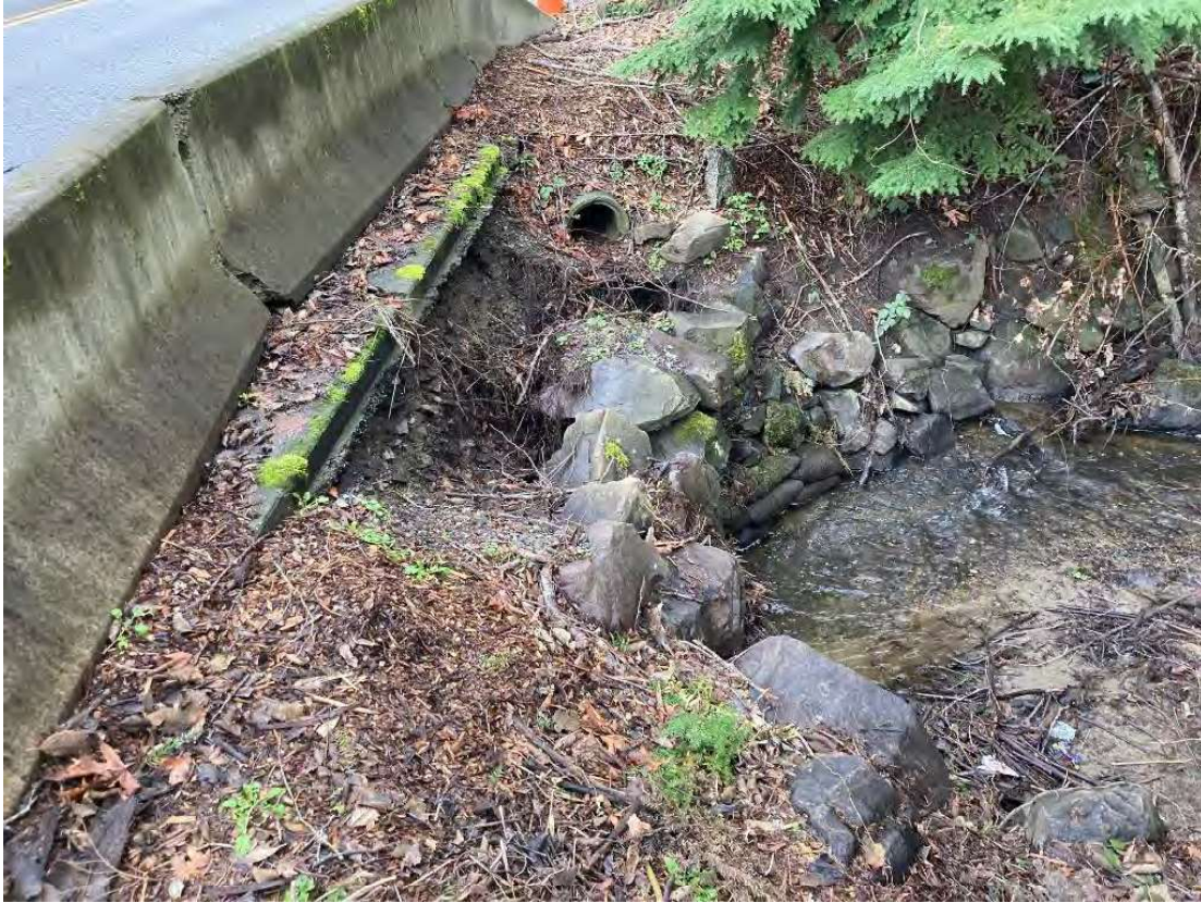
Photo 3. Culvert downstream of property showing storm damage.
