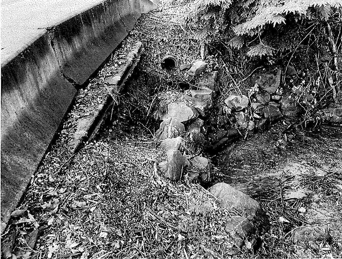
Photo 3. Culvert downstream of property showing storm damage.
